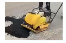
If the pothole is very deep, it is recommended, to apply the product in layers of 5 centimetres at a time to improve compaction with a bigger granulometry at the base (AC-25) and smaller above it (AC-11).
